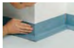
Fix cut-to-measure HSLA skirting in place.
