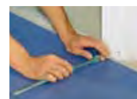
Trace the shape of a doorpost to the linoleum with the help of a scribing bar.
