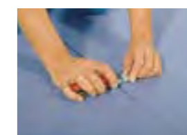
The safest way of cutting a seam: mark the top sheet with an under and over scriber guided along the trimmed edge.
