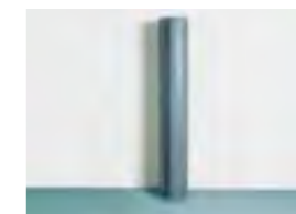
The sheets are cut to size, marked, loosely re-rolled and placed upright to acclimatize to conditions in the room.
