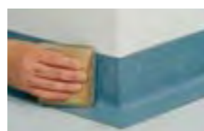
Rub down well to achieve good transfer of adhesive.
