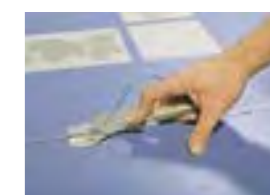
The weld rod is trimmed in two operations, first with the trimming guide fitted, then with the bare blade.
