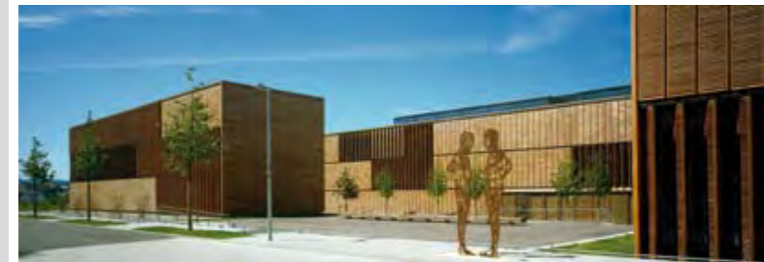
Object: University of Applied Sciences, Aalen Architects: MGF Architekten GmbH, Stuttgart
