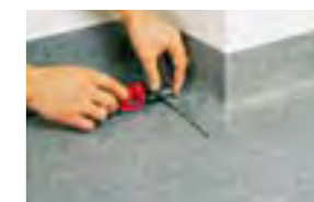
Trimming overlapping strip.
