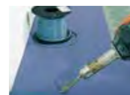
Sealing with a manual hot air gun welder.
