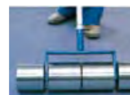
... or with a roller which, due to the gauge of the rollers, exercises sufficient pressure even where slight irregularities occur.
