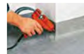
Sealing with weld gun / with colour matching sealing compound
