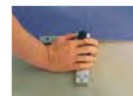
Cutting the first edge of the sheet is best done with a linoleum edge cutter or strip trimmer.
