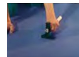
Remaining air bubbles should be rubbed down with an appropriate smoothing tool.
