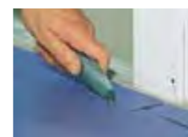
The floor covering is cut along the scored contours.
