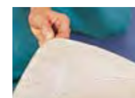
Adhesive must be applied in such a way that the strips of adhesive cover the entire backing of the floor-covering
