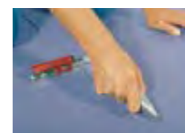
Trimming the top edge with a hooked knife.
