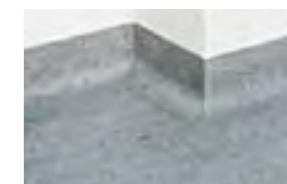
The result: a technically perfect wall join.
