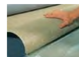
Folding back the trimmed sheets, either half-way back in the case of rooms or lengthways in the case of corridors etc...
