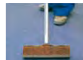
Rubbing down the sheets with a rubbing iron, a device covered with needle felt...
