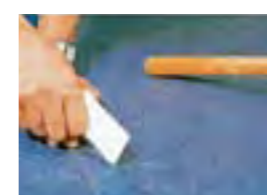
The seam should never fit too tightly. There should be a space of approx. 0.5 mm between adjoining edges when sealing.
